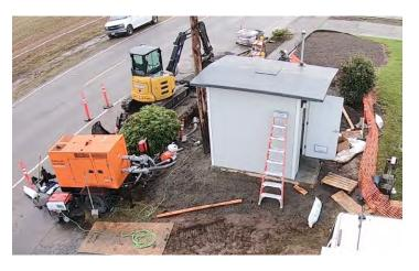
The new pumps are allowing Sublimity to operate at 3.5 horse-power, leaving 6.5 hp untapped until needed. In the coming years, as new homes are added to the city, DPW staff will be able to tap into the additional installed capacity to address future needs without expensive upgrades or retrofits.
